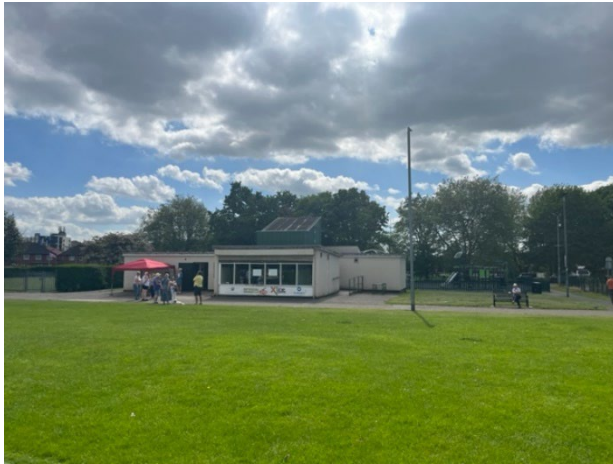
Existing pavilion to be demolished
